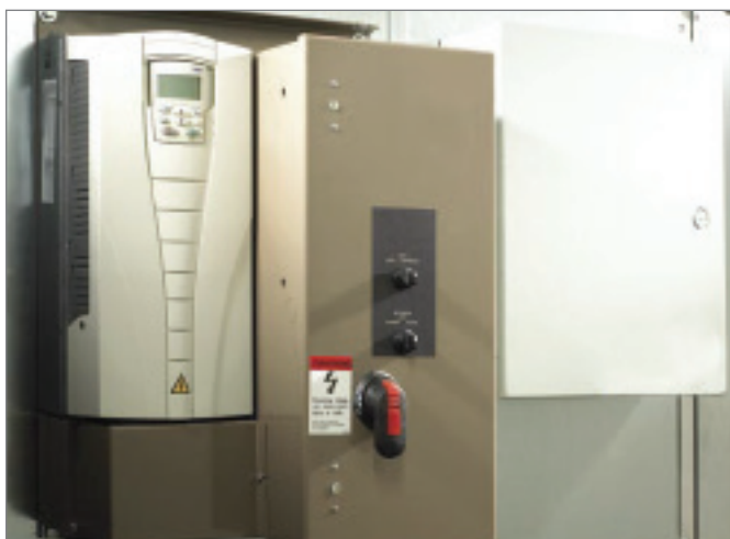
Variable-speed drives offer dramatic fan-energy savings.
