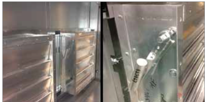
FIGURE 5 - COUNTERBALANCE UNLOCKED FOR START-UP
