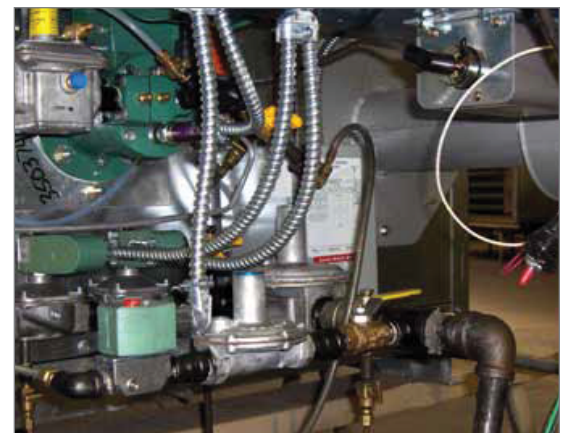
FIGURE 25 - CHECK MAIN GAS SUPPLY PRESSURE
