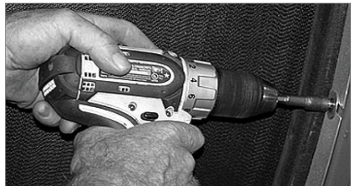
FIGURE 66 - LOOSEN SCREWS BEFORE ADJUSTING SEALS
