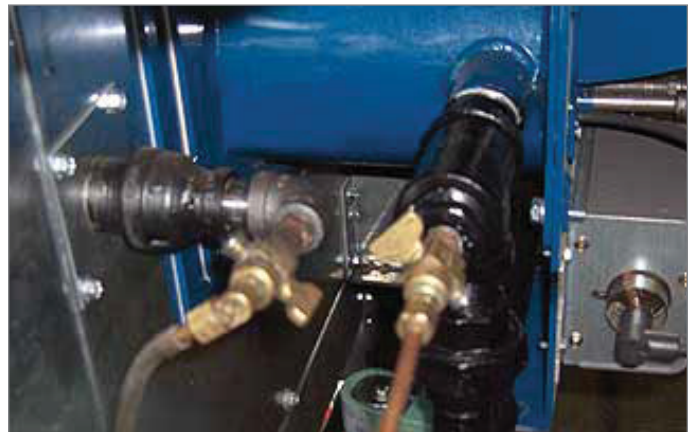
FIGURE 26 - DRAFT OVER FIRE TEST PORT
