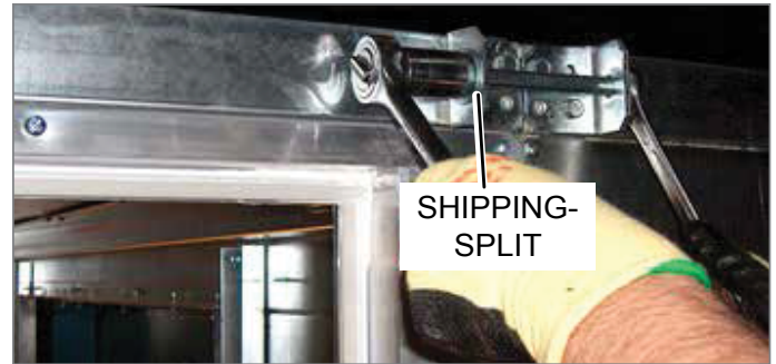
FIGURE 39 - FASTEN BOTTOM LIFTING LUGS
