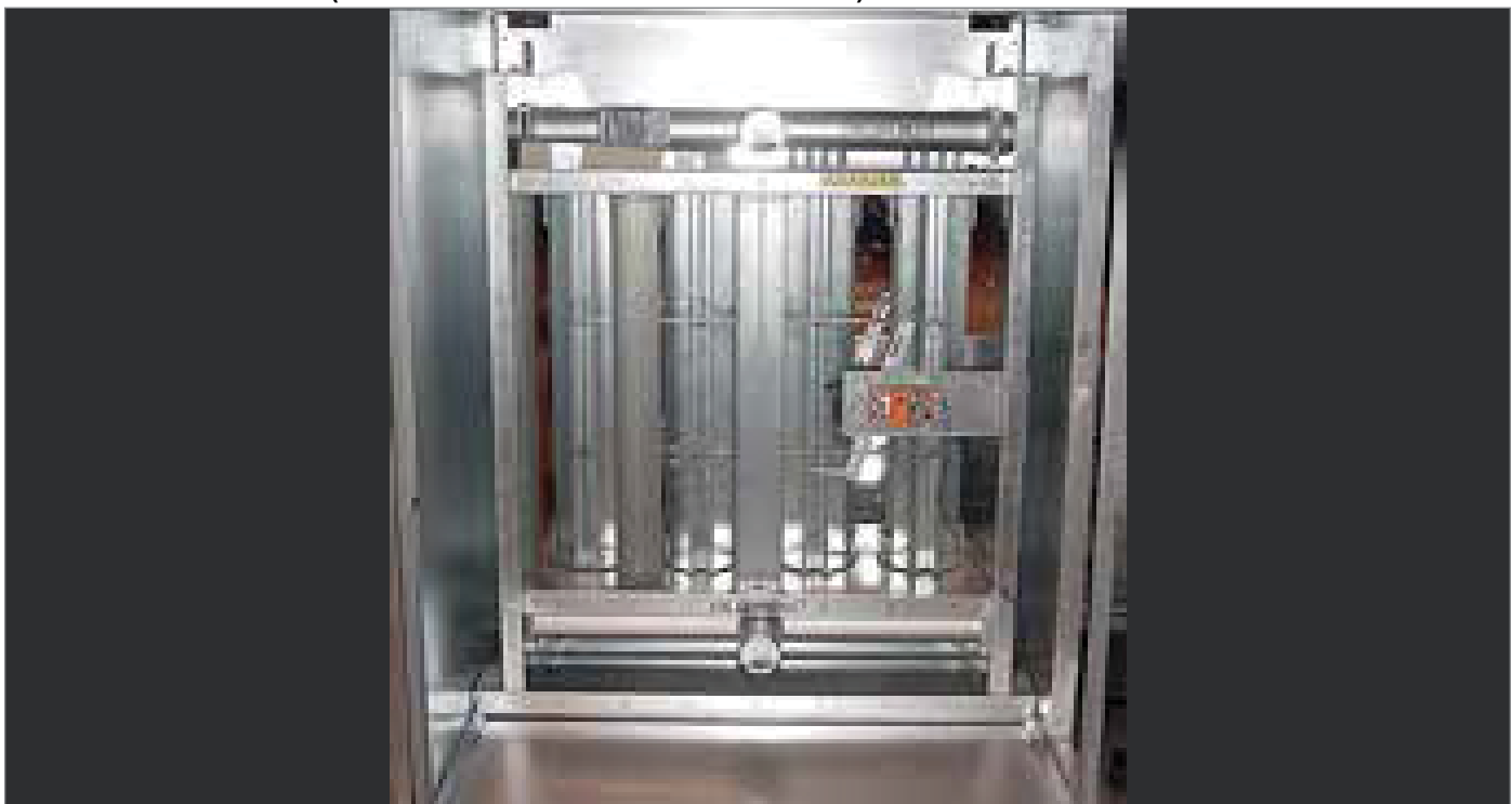
FIGURE 86 - VIFB COIL (FACE-MOUNTED ACTUATOR SHOWN)
