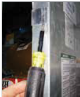
FIGURE 7 - METAL SPACERS ON DOORS
