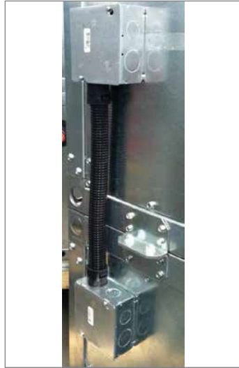
FIGURE 29 - CONDUIT (P/N 025-39024-001) AND SJO CORD (P/N 025-35746-001)
