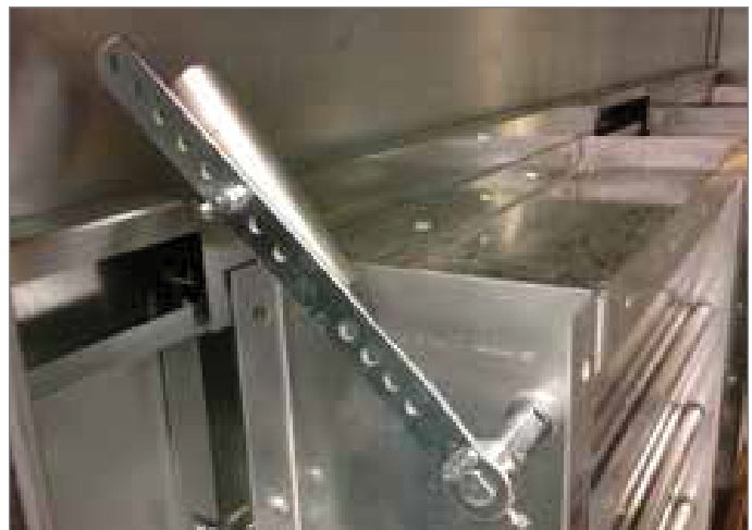
FIGURE 52 - COUNTERBALANCE UNLOCKED FOR START-UP
