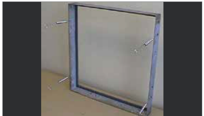
FIGURE 119 - SPRING LATCH PULLED AND FASTENED IN FILTER HOLE
