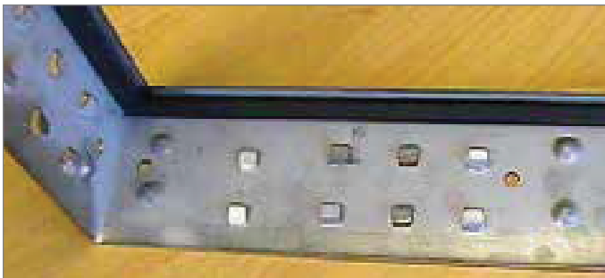
FIGURE 116 - CORRECT USE OF KNOCKOUTS
