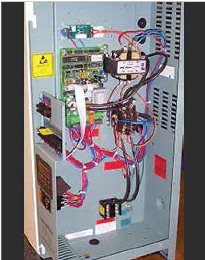
FIGURE 74 - LAYOUT OF TYPICAL HUMIDIFIER PANEL
