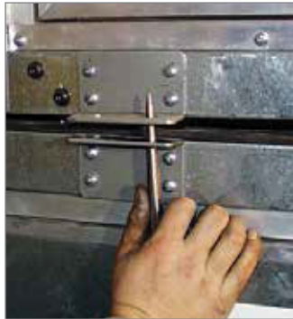
FIGURE 45 - GUIDE BRACKETS TOGETHER
