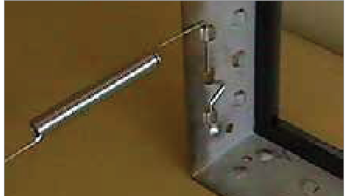
FIGURE 121 - SPRING LATCH PULLED AND FASTENED IN FILTER HOLE
