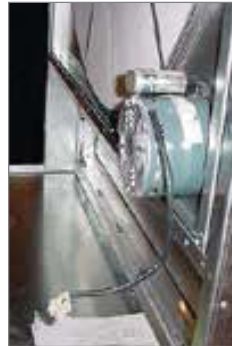
FIGURE 67 - TYPICAL POWER WIRING OF ENERGY RECOVERY WHEEL
