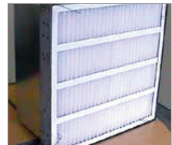
FIGURE 115 - CORRECTLY INSTALLED CARTRIDGE WITH PLEATS
