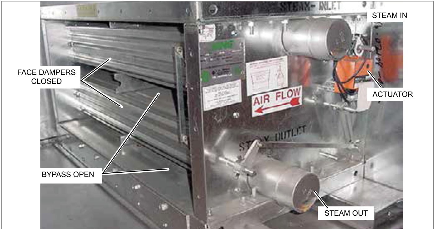
FIGURE 86 - VIFB COIL (FACE-MOUNTED ACTUATOR SHOWN)
