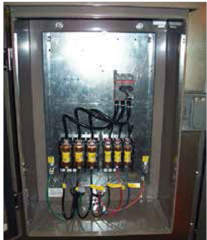
FIGURE 63 - SINGLE POINT POWER CONNECTION
