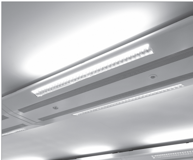
Custom Unit with Integral Lighting Application
