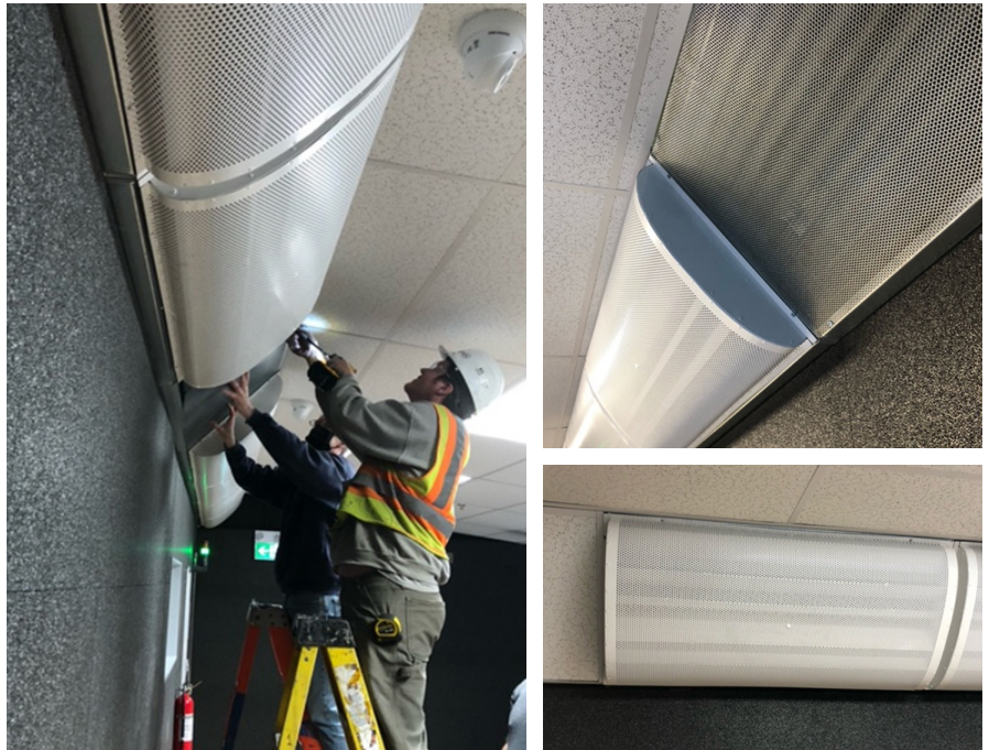
Figure 4: TAD Installation Photos
