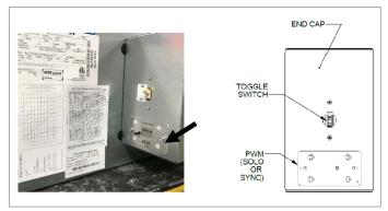
FIGURE 1 – PWM Installed in Enclosure (example installation location)
